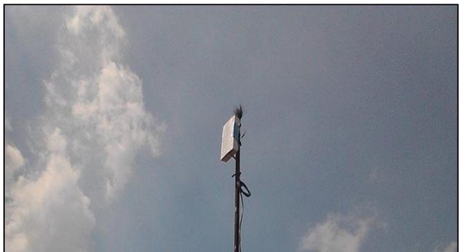
On base station side, a WBS is usually installed using a special bracket or signal tower due to the large size of the Sector Antenna. The Pharos Sector Antenna is designed with a dedicated slot to affix a WBS. You should fix the antenna to the signal tower with a metal bracket. For detailed information, please refer to the [TL-ANT5819MS Installation Guide](#).
