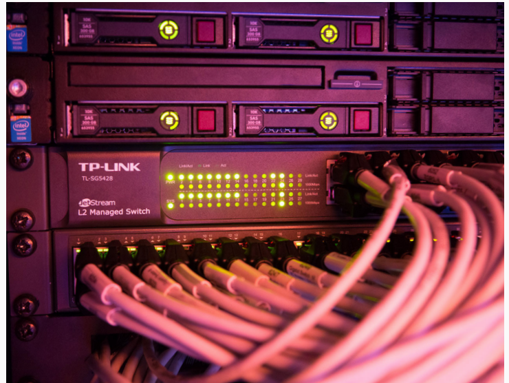
TL-SG5428 in use within picture and sound range in the broadcasting van.
