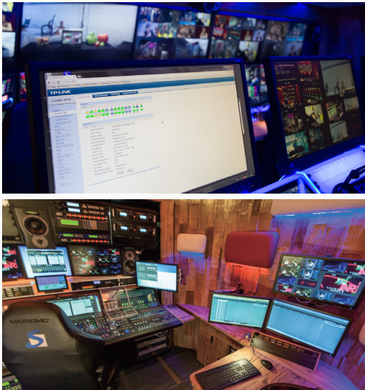
Full data coverage within two main switches. (Source: TV Skyline)
